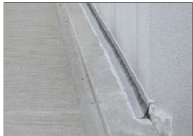
Angled installation with pre-assembled shaped part
