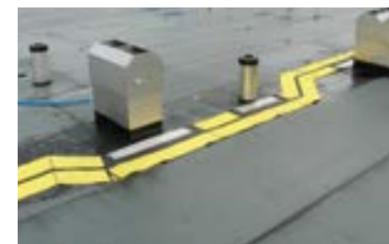
Enclosures can easily be vulcanized into the FlamLINE® expansion joint strip.
