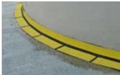
Consistent FlamLINE® joint seal over a number of corners and levels.
