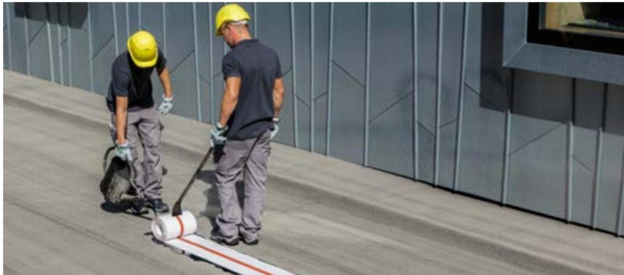
RedLINE® expansion joint strips are generally delivered prefabricated with all preforms on a project-specific basis. For installations in several stages or for very long building joints that make handling more difficult, the specially developed vulcanization device can be used to produce the strip on site. Ask our technical services department directly about the options available ([info@soba-inter.com](mailto:info@soba-inter.com)).
