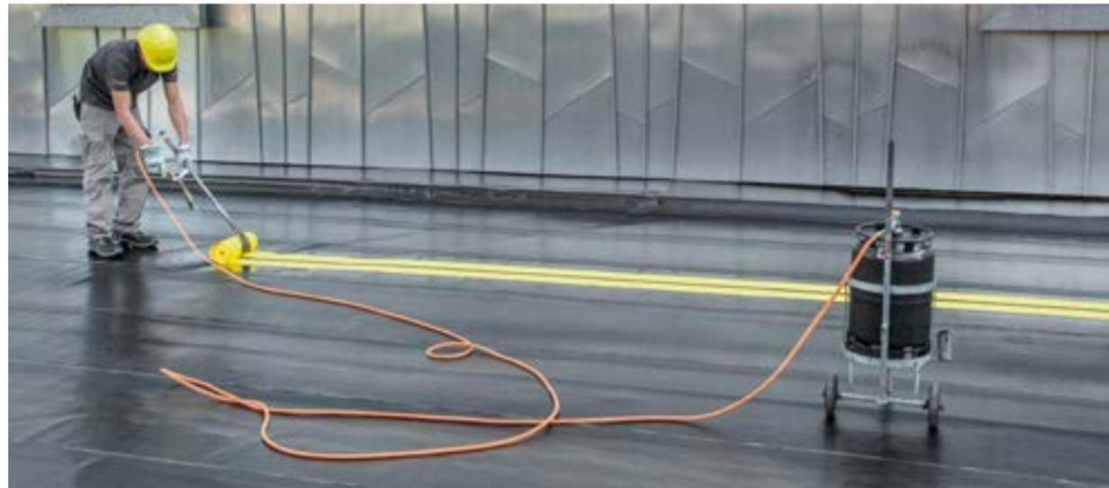
FlamLINE® expansion joint strips are generally delivered prefabricated with all preforms on a project-specific basis. For installations in several stages or for very long building joints that make handling more difficult, the specially developed vulcanization device can be used to produce the strip on site. Ask our technical services department directly about the options available ([info@soba-inter.com](mailto:info@soba-inter.com)).
