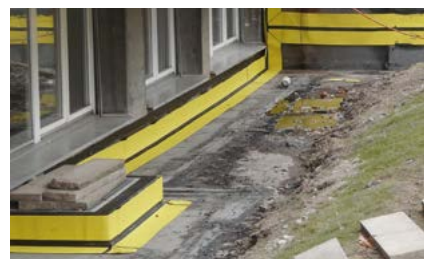
Consistent FlamLINE joint seal over a number of corners and levels.
