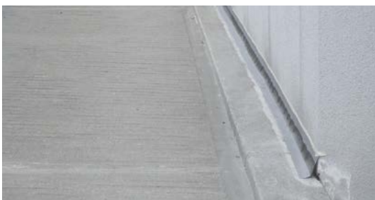
Direct gluing of the joint tape to the concrete surfaces.
