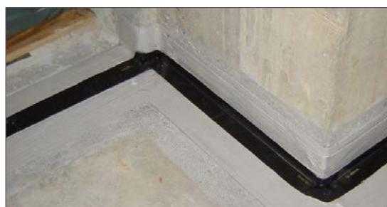
Angled installation with prefabricated form piece.
