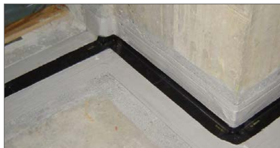
Angled installation with prefabricated form piece.
