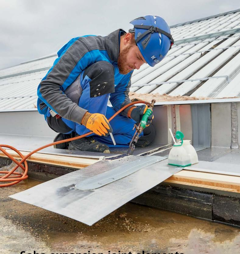
Soba expansion joint elements for optimal movement compensation
